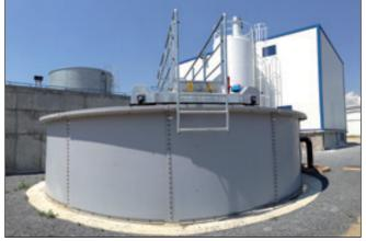
2m high W-Tank® settling tank.
