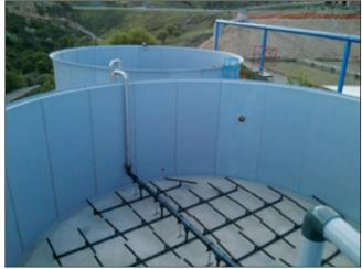
Two 5m high W-Tank  $^{\otimes}$  storage tanks with a diameter of 13.2m and a volume of  $684m^3.$
