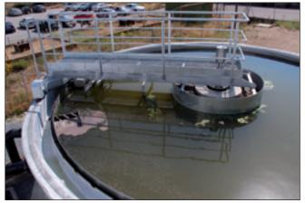
W-Tank® settling tank.
