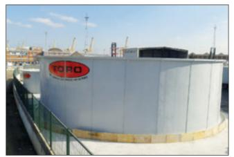
5m high W-Tank^ $\otimes$  storage tank with a volume of 993m³ and 3m high W-Tank^ $\otimes$  storage tank with a volume of 126m³.
