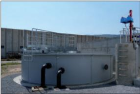
Settling tank and connections.
